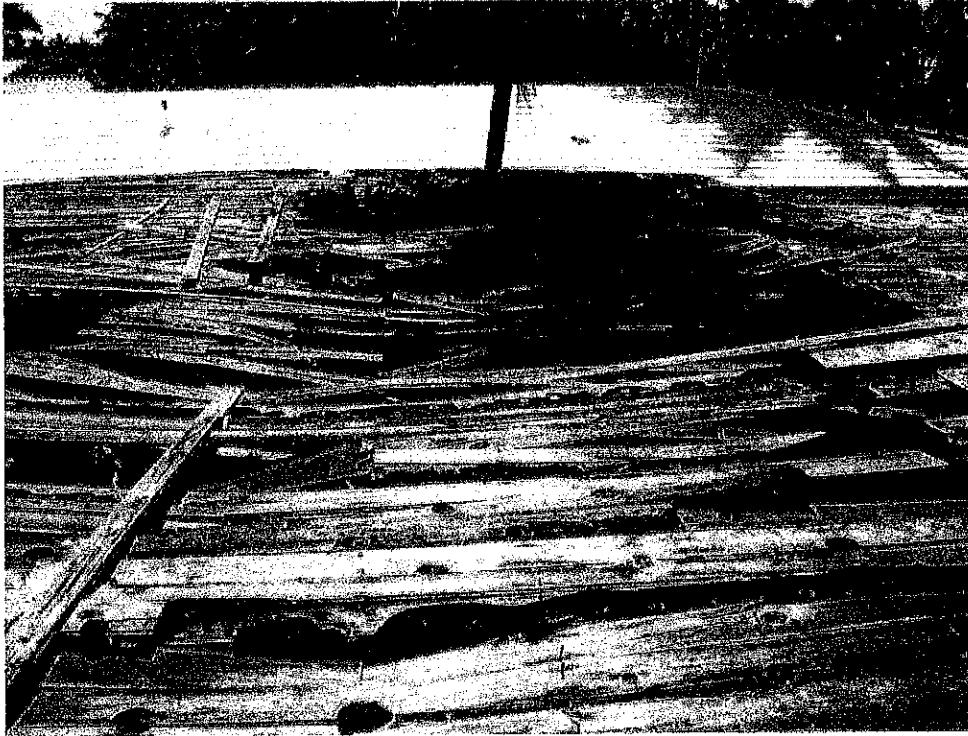
Photograph 1: Overview of Roof Deterioration
