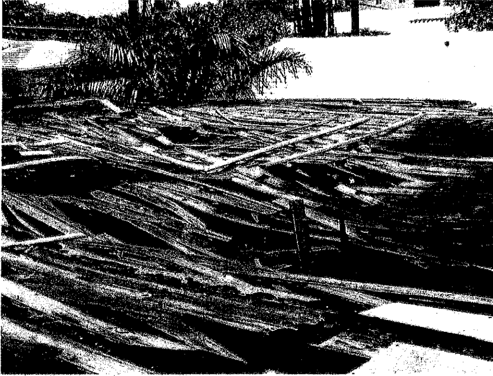
Photograph 3 – Deterioration of Roof and Interior Walls
